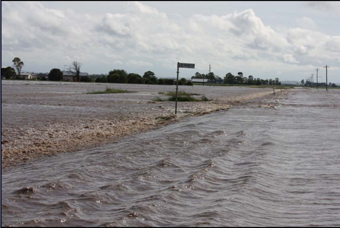
Flood water rushing across the Gore Highway in December 2010.
